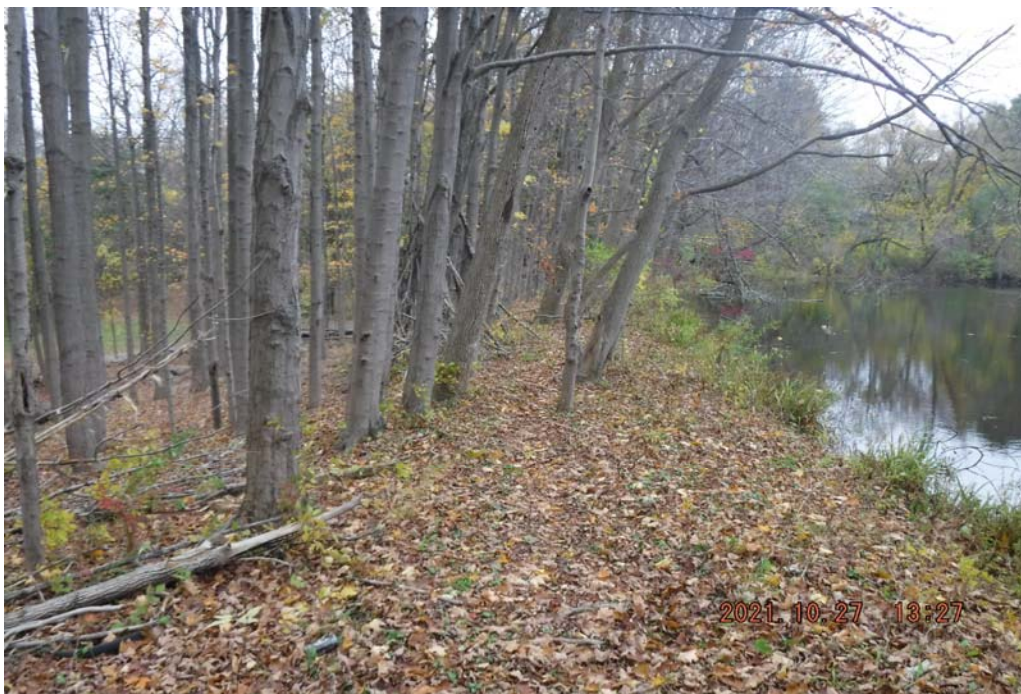
Photo 6 Dam ID# 195-1592 Sky View Pond Dam 10/27/2021 Dam crest View looking right from service spillway
