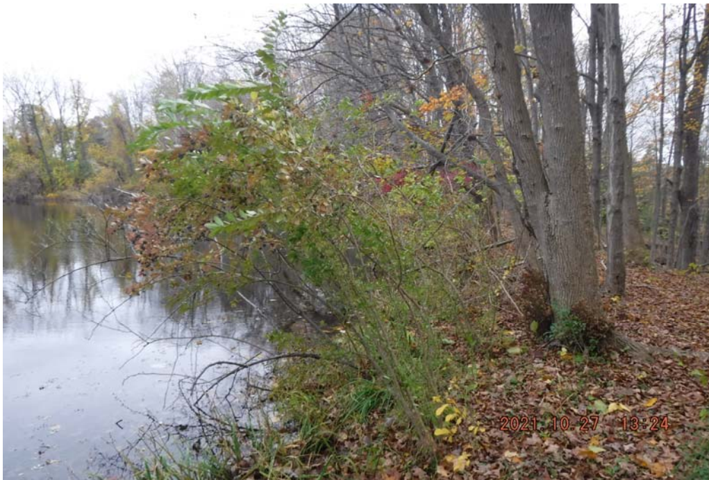
Photo 2 Dam ID# 195-1592 Sky View Pond Dam 10/27/2021 Upstream slope View looking left from right end of dam
