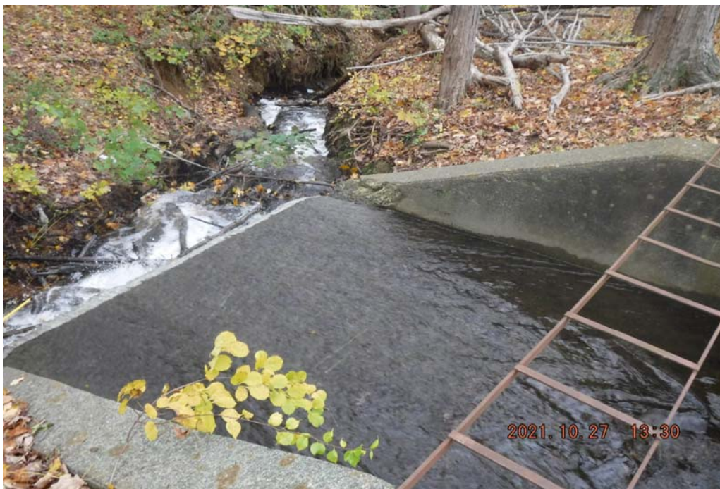
Photo 10 Dam ID# 195-1592 Sky View Pond Dam 10/27/2021 Service spillway outlet slab and drop-off View looking right from left side
