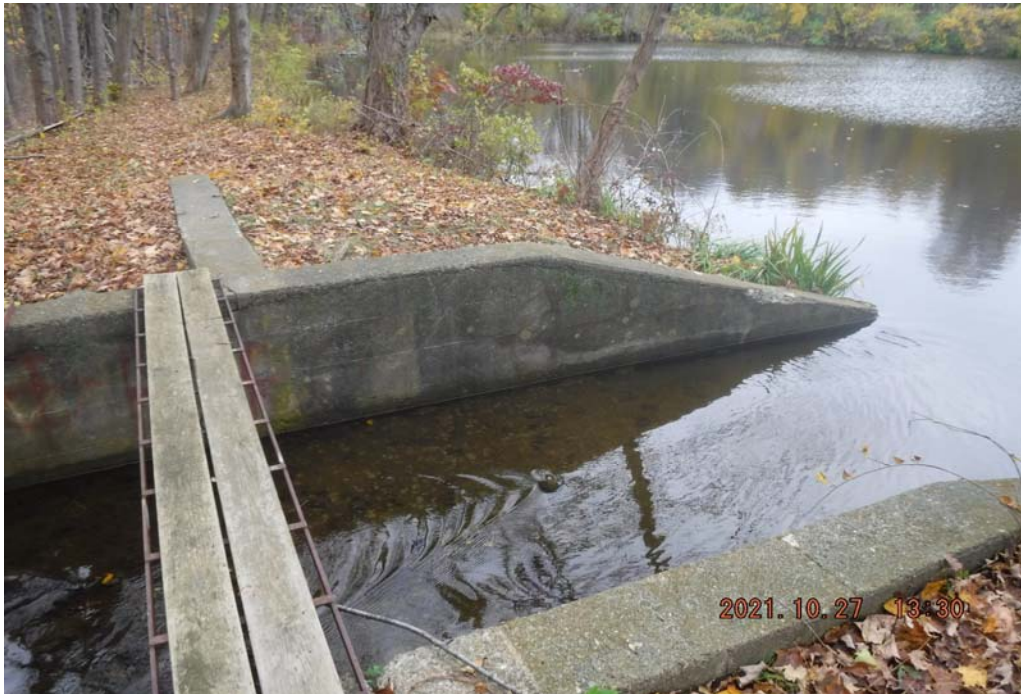
Photo 9 Dam ID# 195-1592 Sky View Pond Dam 10/27/2021 Service spillway upstream entrance View looking right from left side
