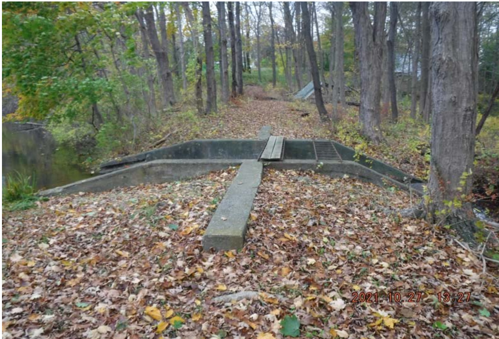
Photo 7 Dam ID# 195-1592 Sky View Pond Dam 10/27/2021 Service spillway towards left end of dam View looking left from right side
