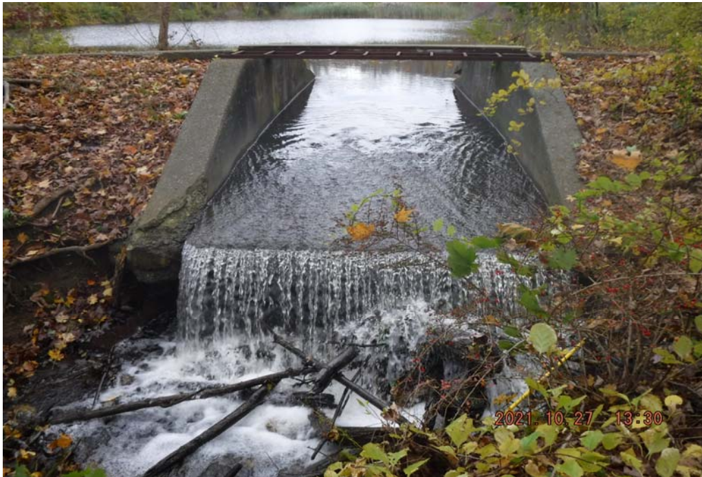
Photo 11 Dam ID# 195-1592 Sky View Pond Dam 10/27/2021 Service spillway View looking upstream from outlet channel
