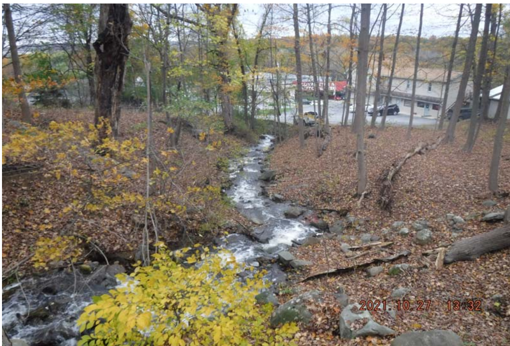
Photo 14 Dam ID# 195-1592 Sky View Pond Dam 10/27/2021 Service spillway downstream outlet channel View looking downstream
