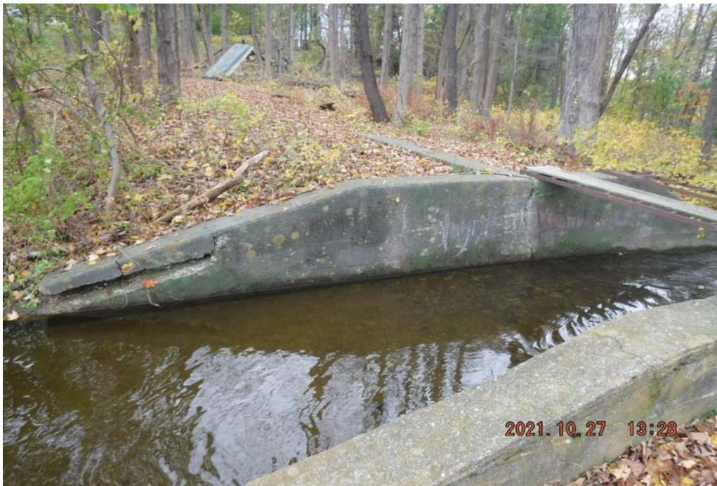
Photo 8 Dam ID# 195-1592 Sky View Pond Dam 10/27/2021 Left spillway side wall View looking left from right side
