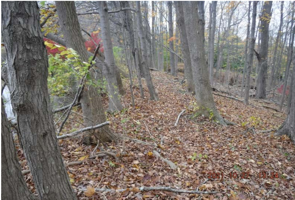
Photo 1 Dam ID# 195-1592 Sky View Pond Dam 10/27/2021 Right end of dam crest View looking left from right end of dam
